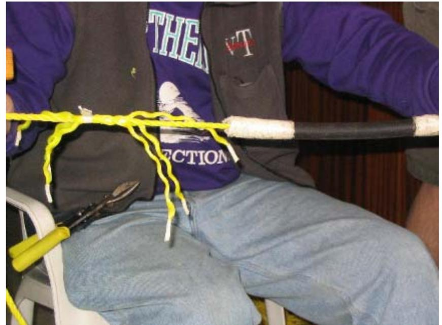
**Figure 12 – Ropes Mated, Tube Ready to Slide Over Splice**
